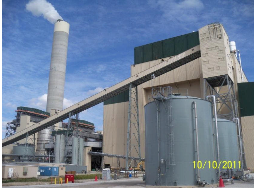
Unit 1 Generating at 30 MW
