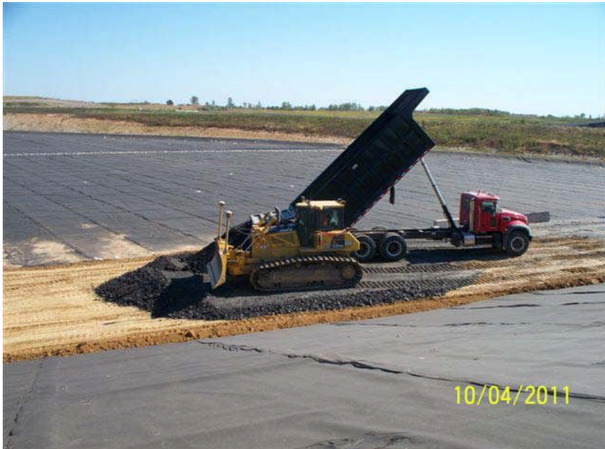
Placing Mine Residue at Jordan Grove Disposal Area
