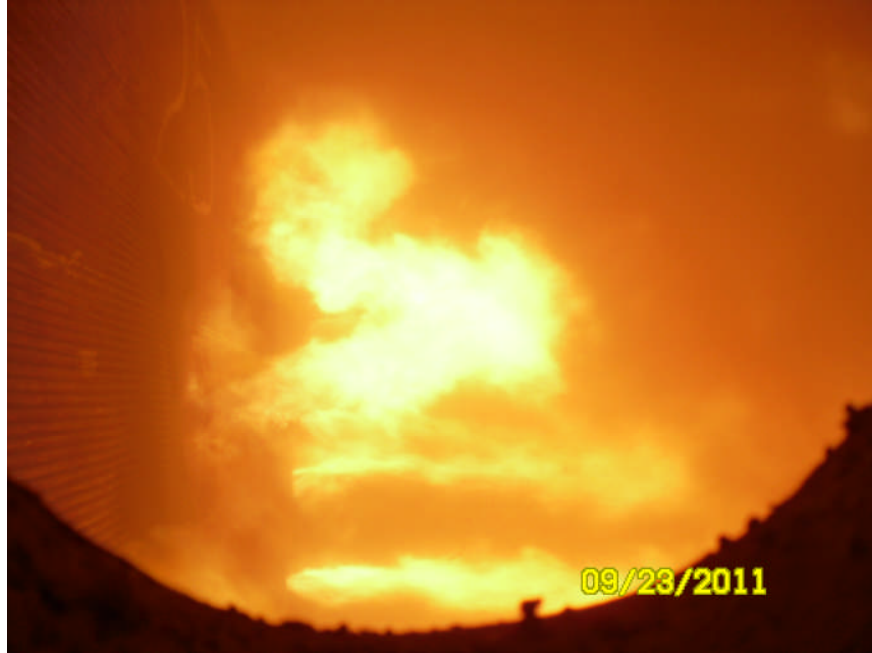
Unit 1 Boiler Coal Firing
