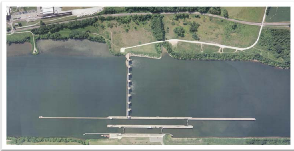
Willow Island Locks & Dam prior to start of construction
