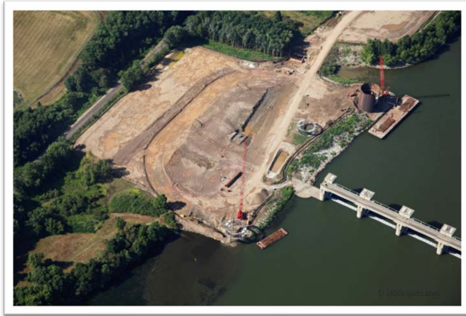
Willow Island construction July 2011
