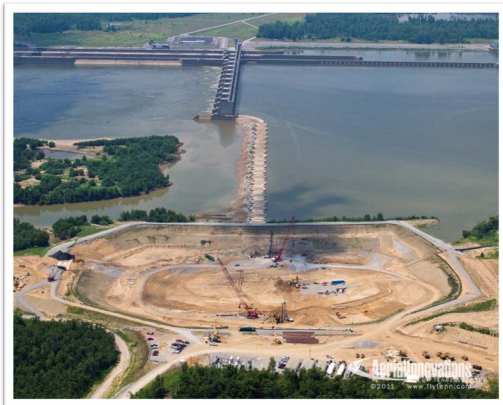
Smithland construction July 2011
