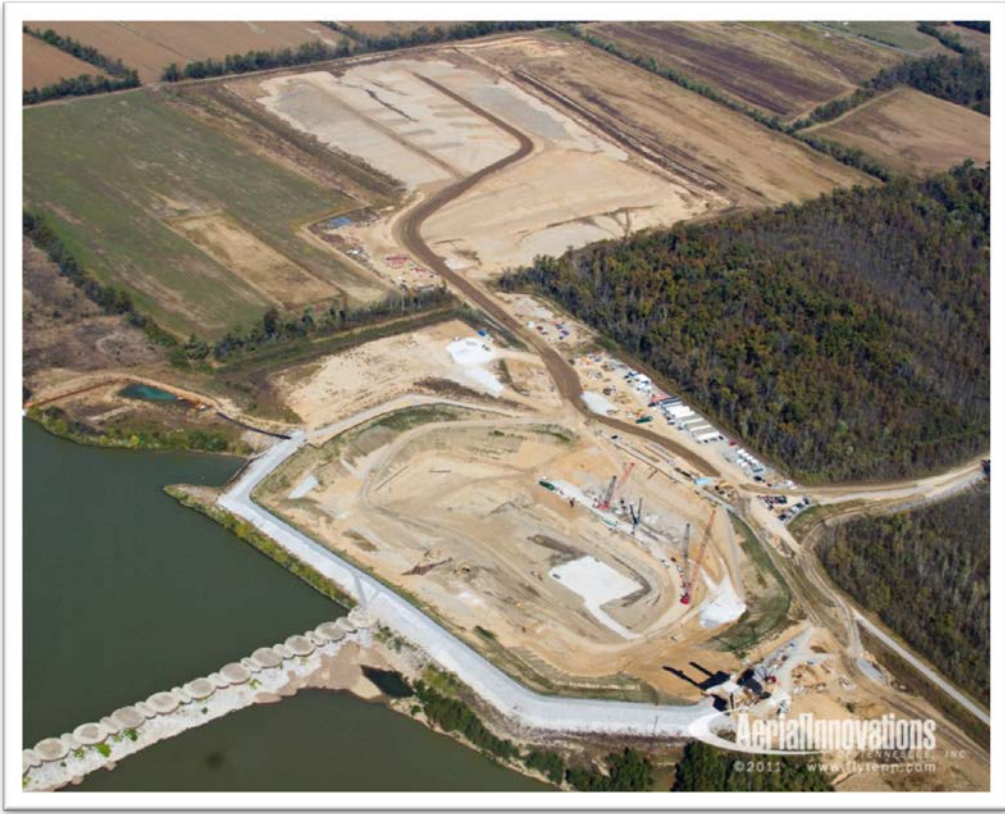
Smithland construction October 2011
