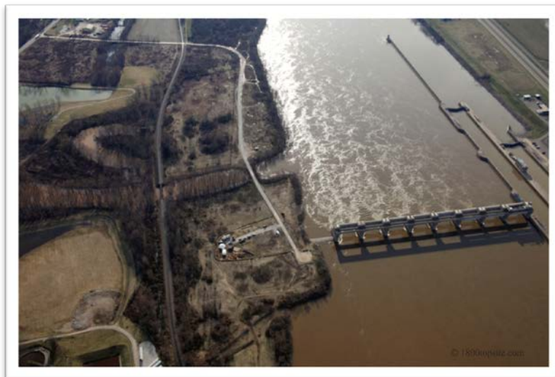
Willow Island construction March 2011
