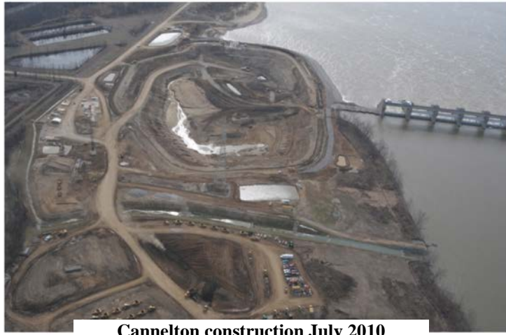
Cannelton construction July 2010
