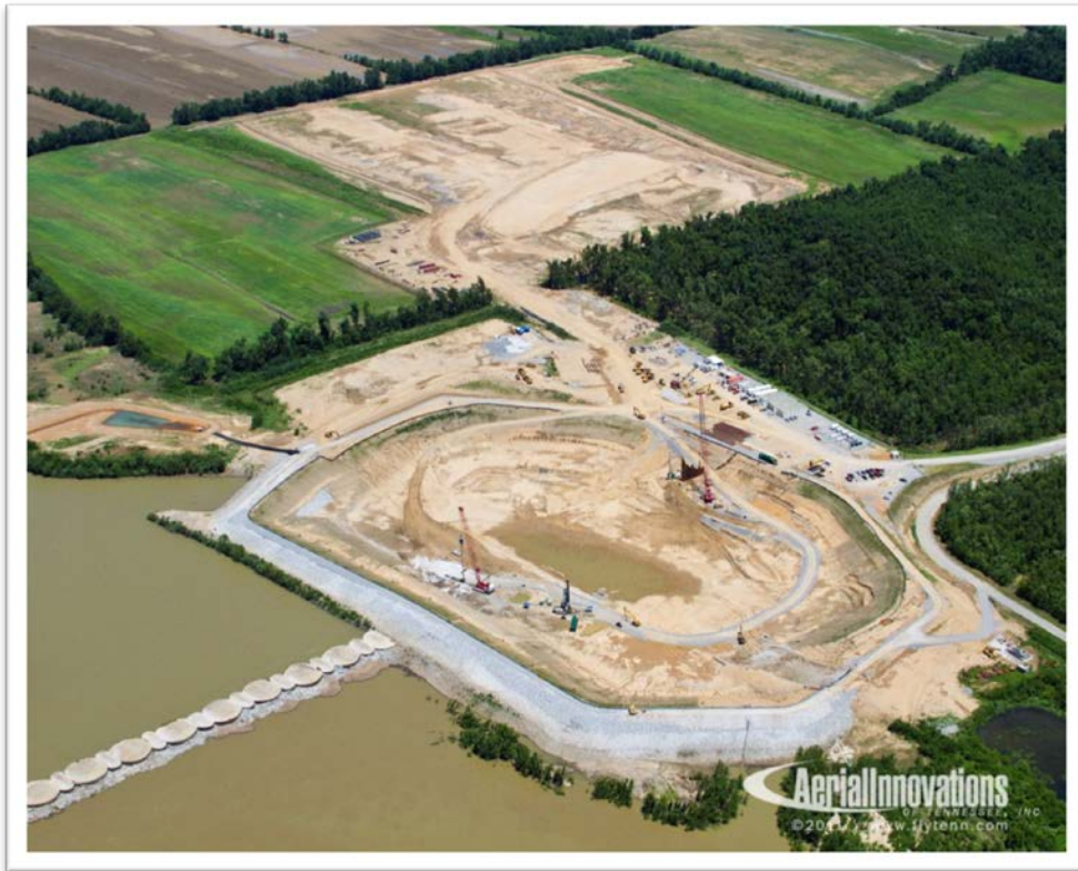
Smithland construction June 2011
