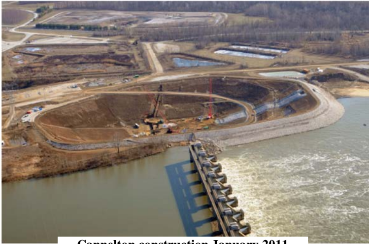
Cannelton construction January 2011
