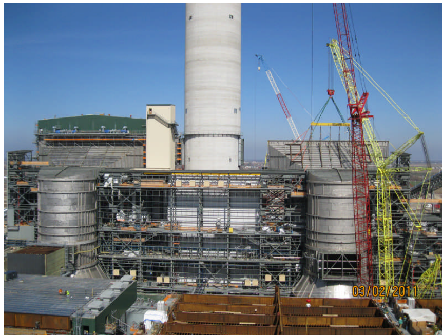
Air Quality Control System Construction
