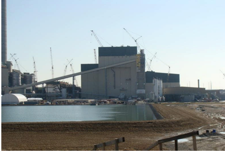
Power Plant West View
